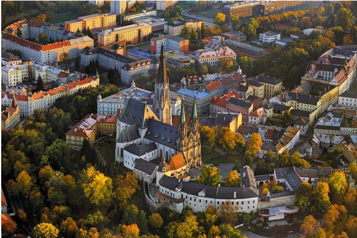
A view of Saint Wenceslas Cathedral with the Palacký University Faculty of Education building in the background.
